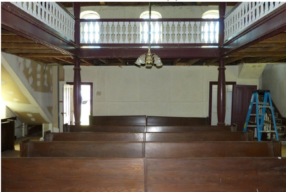
Photo 19 – First floor, nave
