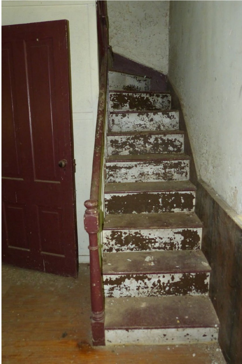
Photo 23 – First floor, stairway to gallery
