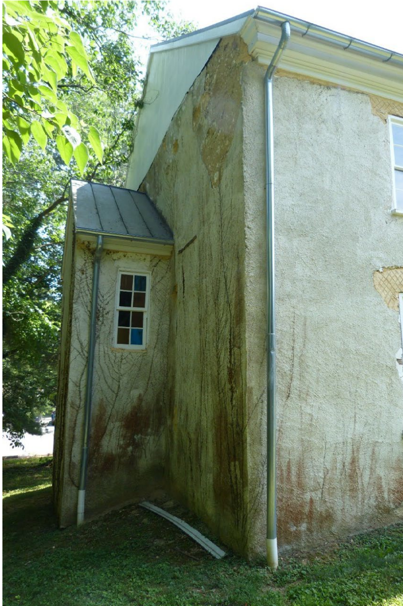
Photo 3 – North and East elevations
