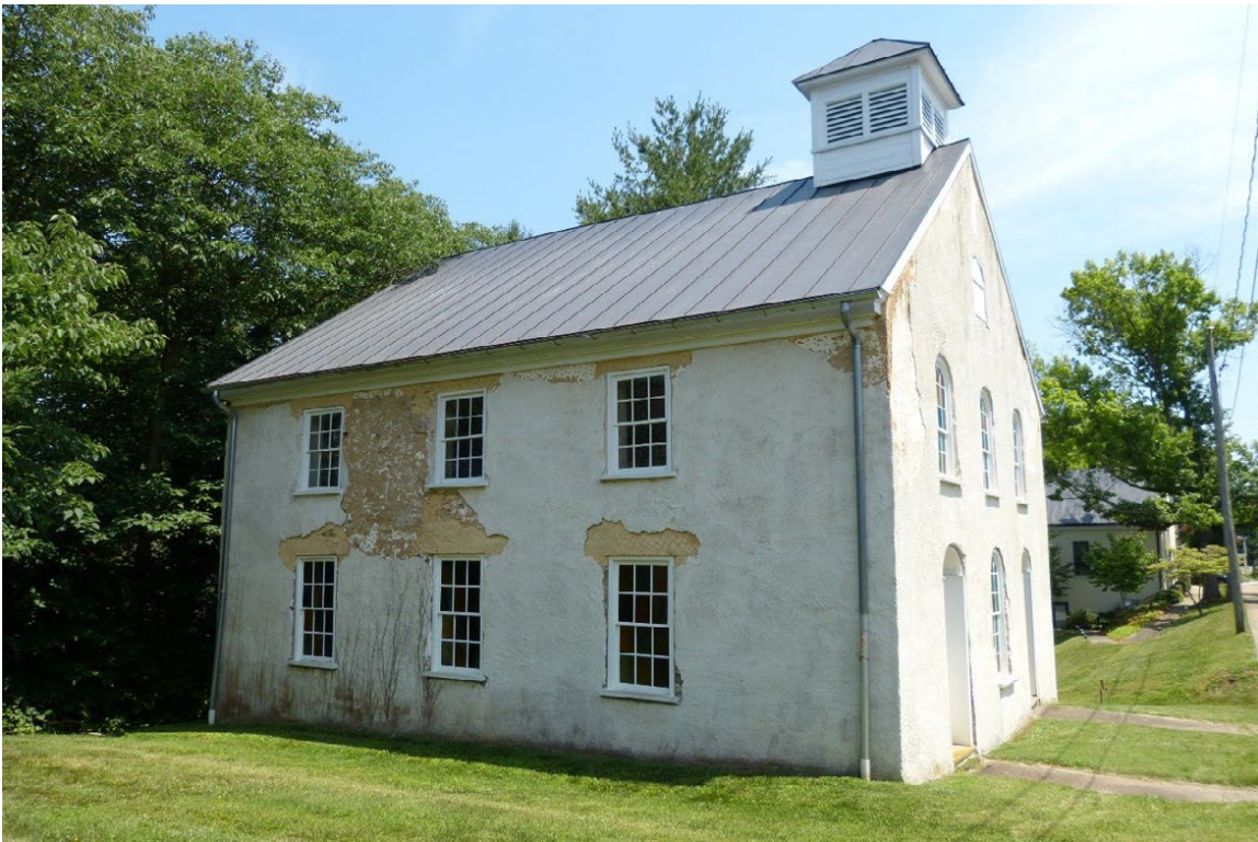
Photo 2 – North and West elevations
