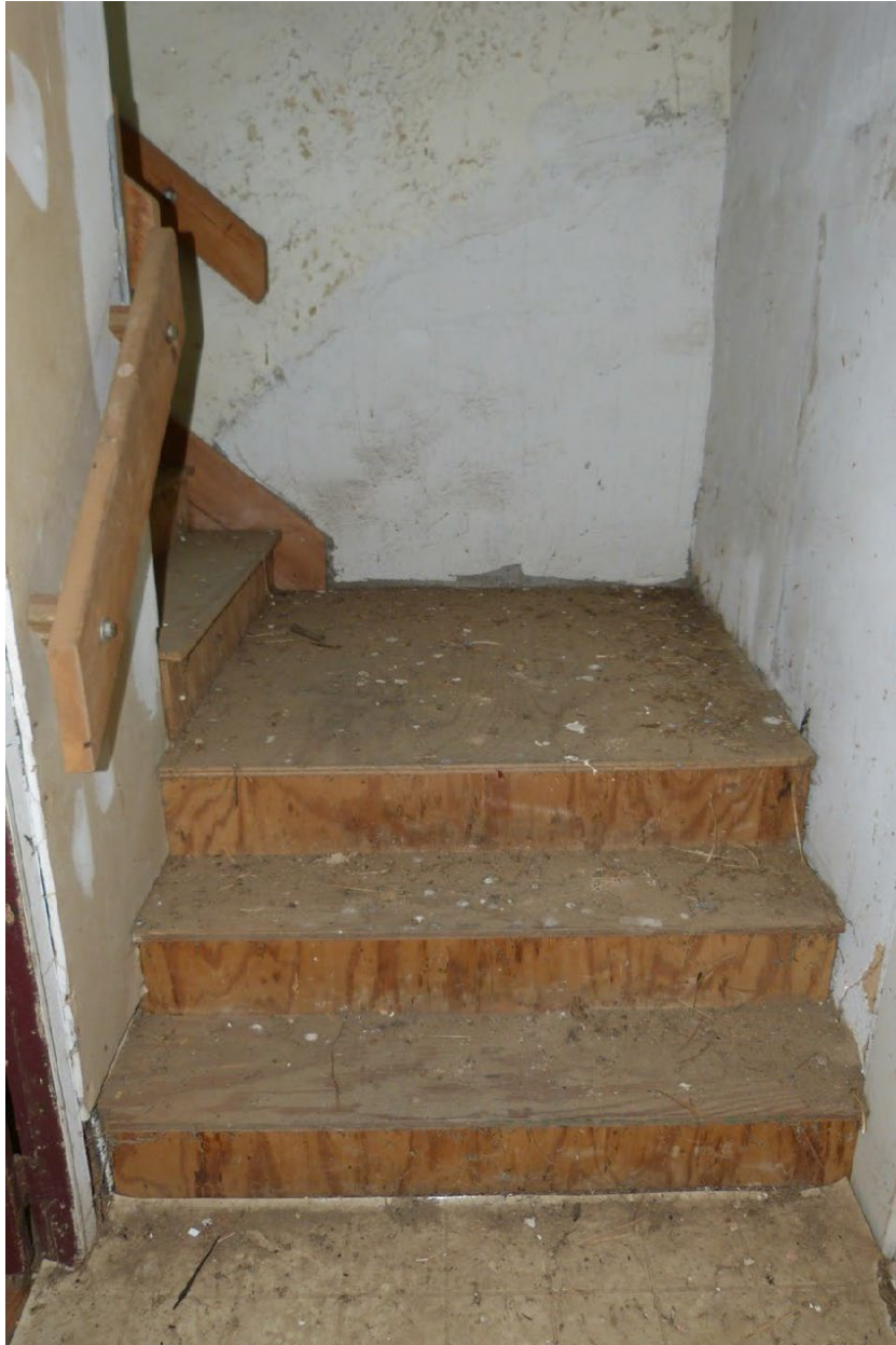
Photo 15 – First floor, stairway to gallery
