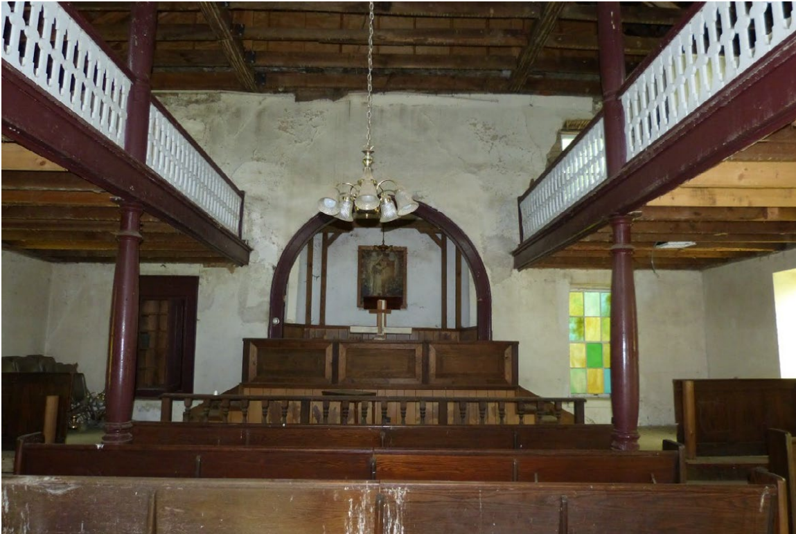
Photo 20 – First floor, nave
