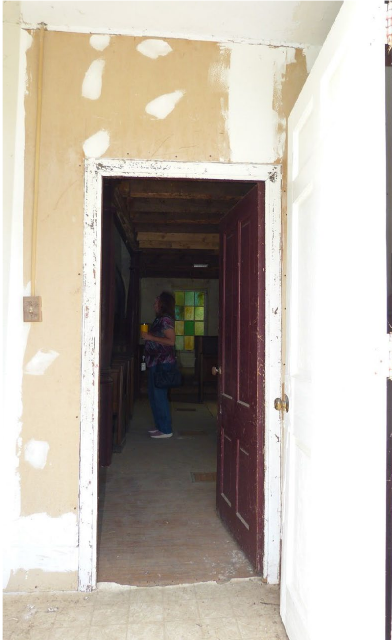
Photo 12 – First floor, entryway
