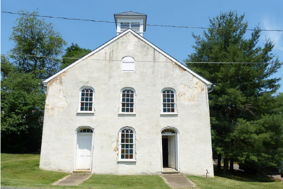
Photo 1 – Façade, West elevation
