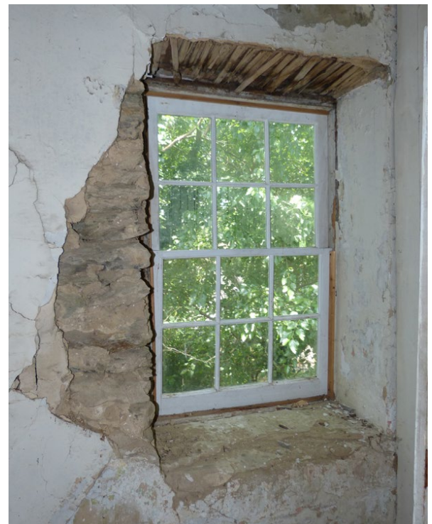
Interior Wall and Window Opening Detail, CPG, July 2024
