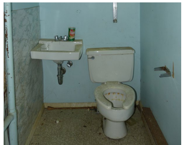
First Floor Bathroom, CPG, July 2024
