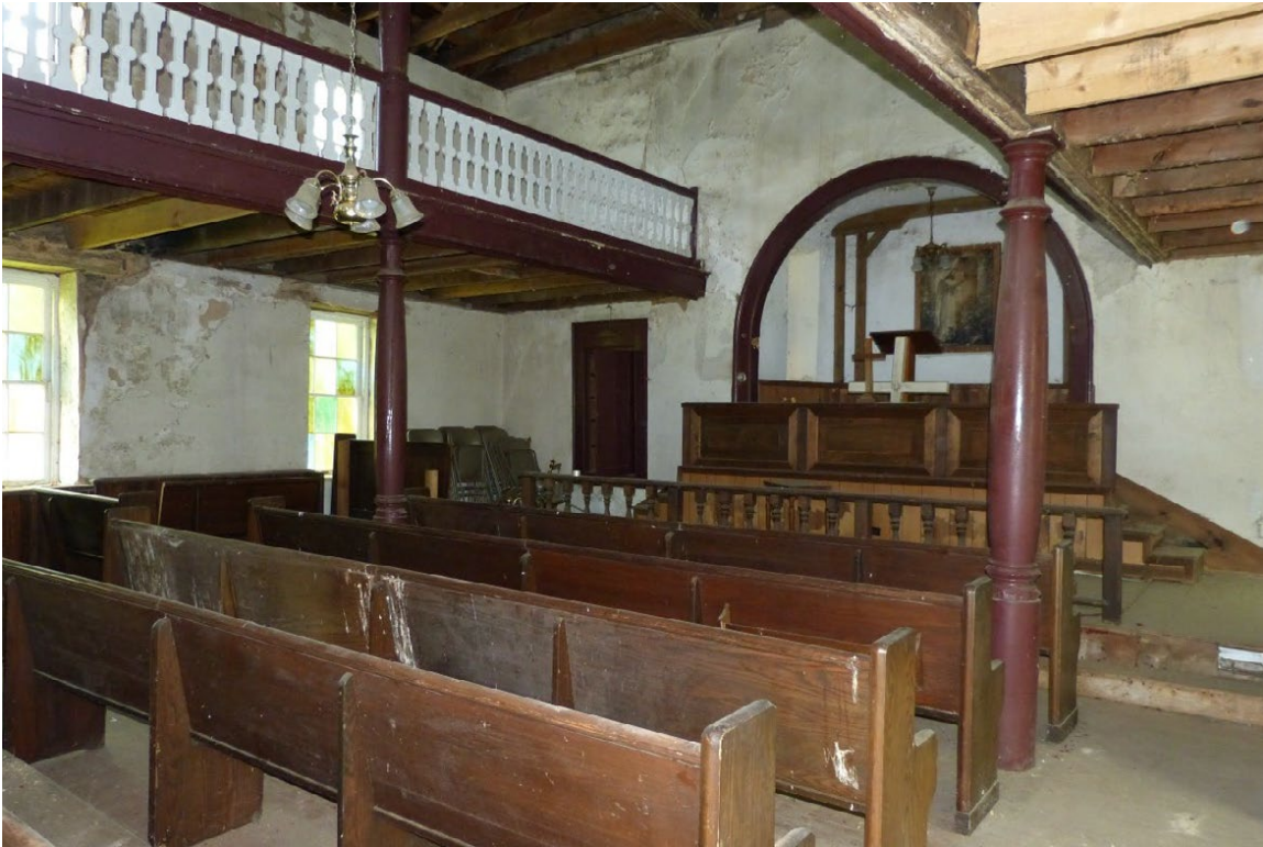
Photo 16 – First floor, nave
