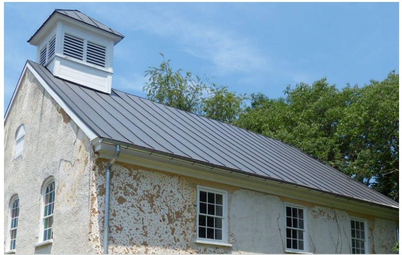
Roof Detail, West and South Elevations, CPG, July 2024
