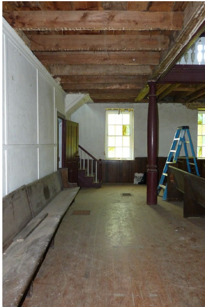
Photo 17 – First floor, nave
