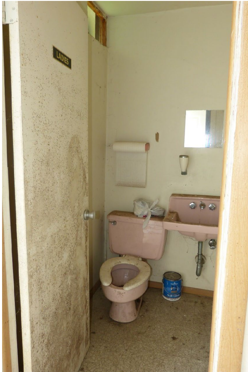
Photo 14 – First floor, bathroom
