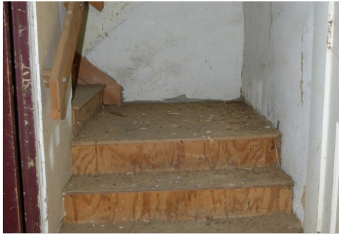
First Floor, Stairway to Gallery, CPG, July 2024
