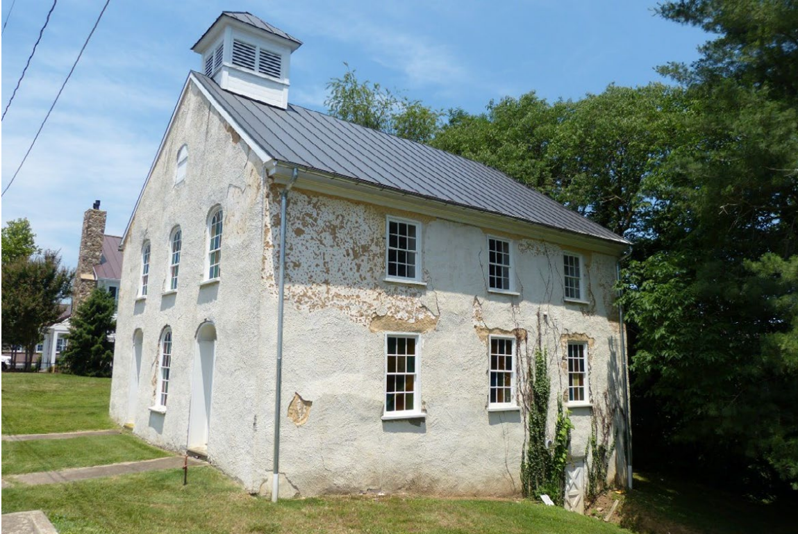
Photo 6 – West and South elevations
