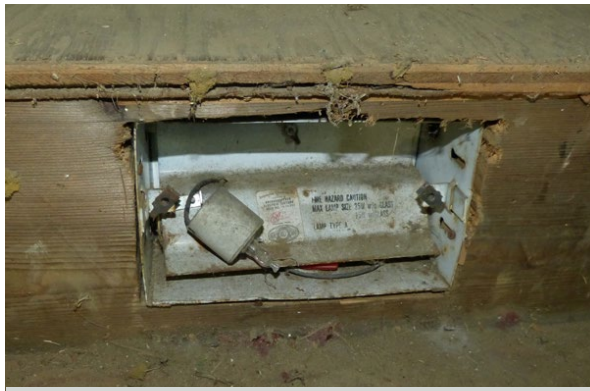
Light Fixture Detail, CPG, July 2024
