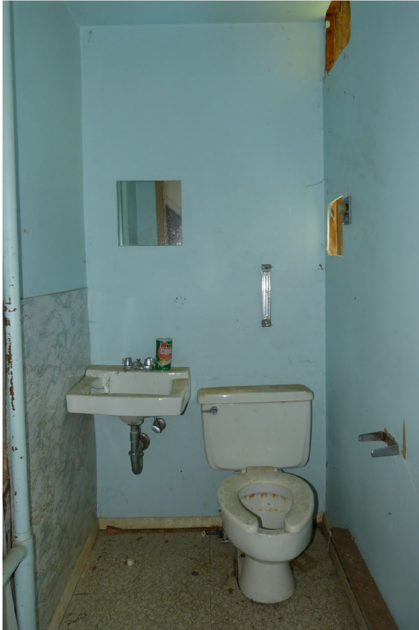
Photo 22 – First floor, bathroom
