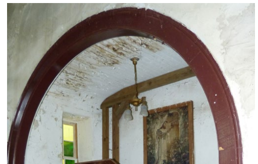
First Floor Pulpit Ceiling Detail, CPG, July 2024
