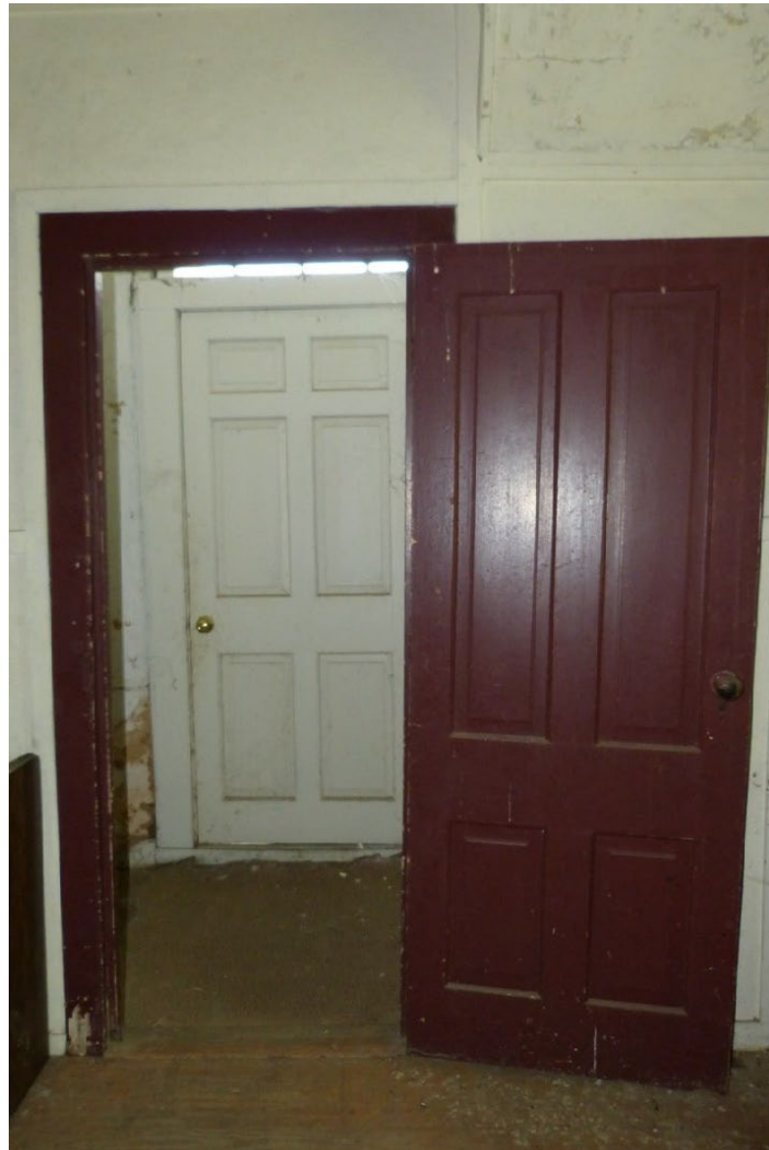
Photo 21 – First floor, entryway
